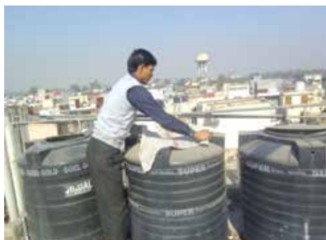
Overhead water tanks
